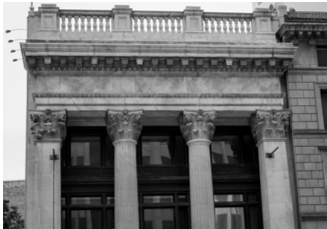
The Bank of Toronto Building at 456 Main Street (now the Fox and Fiddle) with two fluted Corinthian columns included between unfluted Corinthian pilasters
